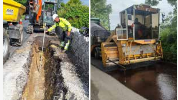
Site Foreman using a laser level for Drainage works on the R-352 at Clooney
