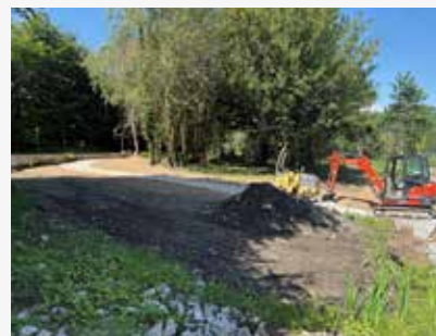
Topsoiling verges at Tobermurragh paths
