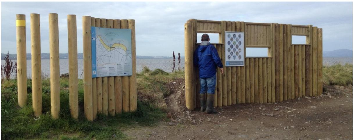
Where birds are already used to people or where only minimal screening is needed, the screens can act to signify the right place to view from and also provides a platform for interpretation. In such an exposed site this type of construction is extremely robust to high winds.
