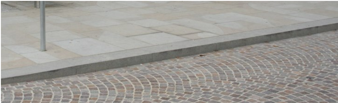
Granite kerbing delineates edgeways and creates a crisp roadside edge. Granite kerbing has the ability to work well with a variety of materials
