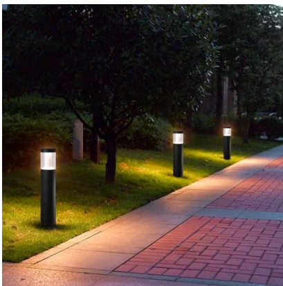
Bollard Lighting is less intrusive than traditional pole lighting and contributes to more intimate spaces that do not obstruct views of important Architecture/built heritage. Bollard lighting provides a localised area of luminosity.
