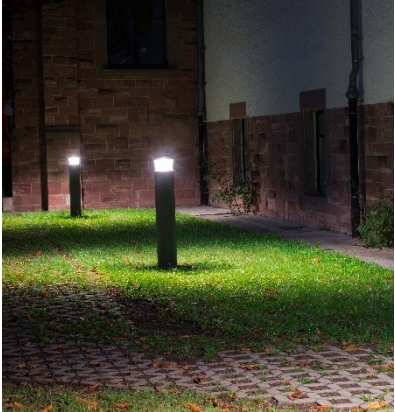
Bollard Lighting is less intrusive than traditional pole lighting and contributes to more intimate spaces that do not obstruct views of important Architecture/built heritage. Bollard lighting provides a localised area of luminosity.
