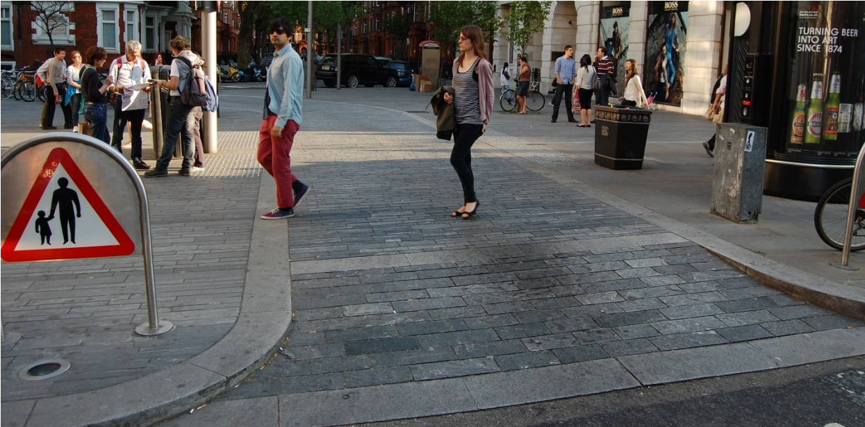
Kilkenny Blue Limestone Paving and Granite Kerbs to a shared Space crossing point
